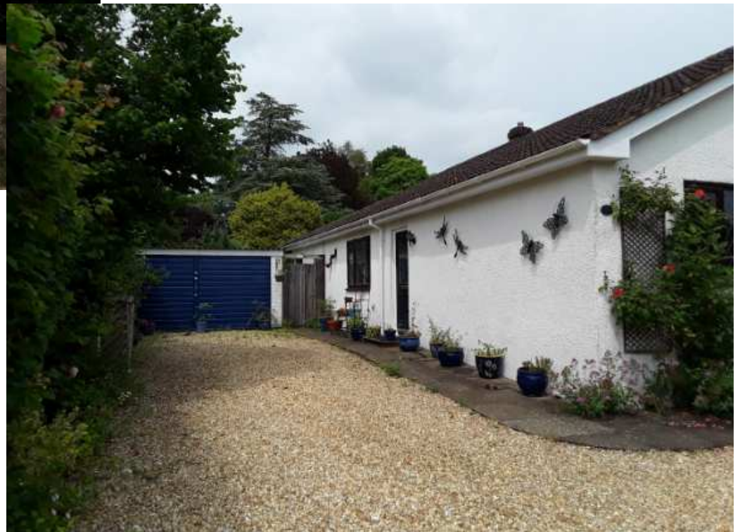
Front of existing dwelling looking North
