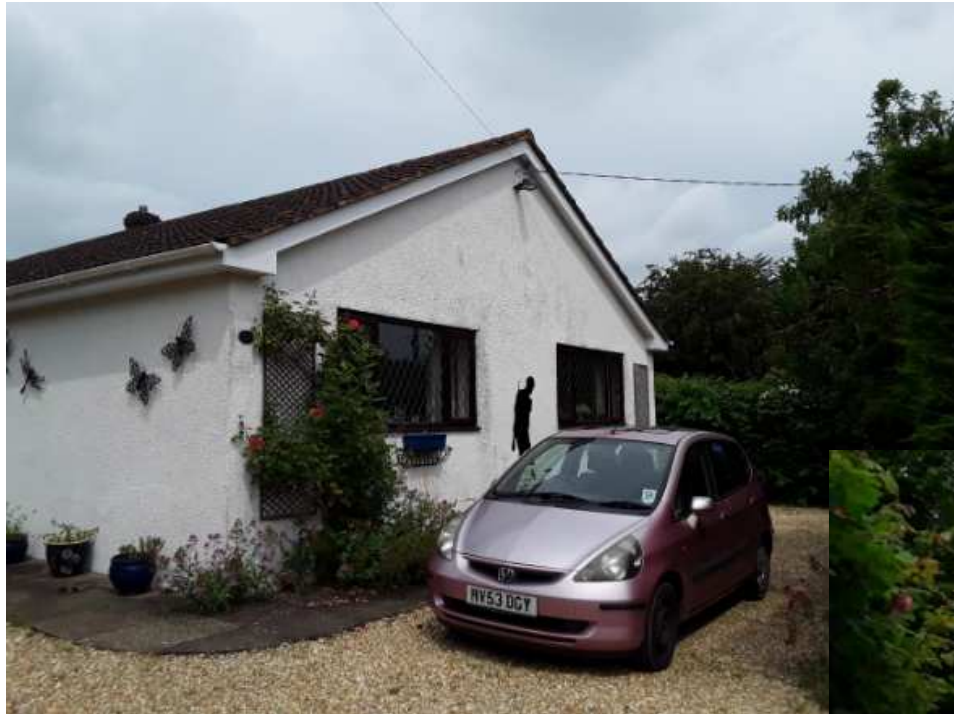
Front of existing dwelling looking North East
